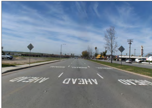
Portions of Alessandro Boulevard are exceptionally wide discouraging walking, biking, and pedestrian activity.
