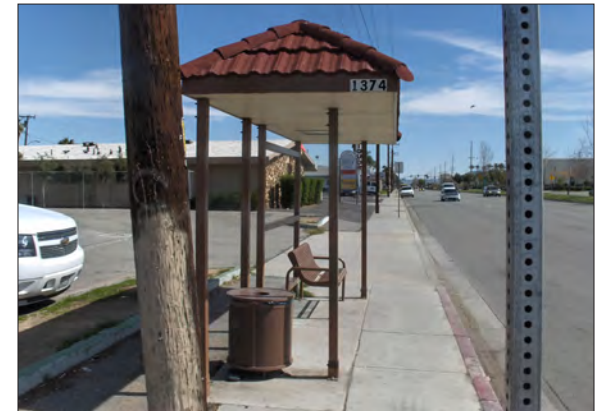
A bus stop with benches and a shade structure invites riders along the Alessandro Boulevard corridor.
