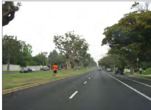
San Vicente Boulevard: 35 to 40 miles per hour, 2 lanes each direction, parallel parking, large planted median, class 2 bike lane, primarily residential
