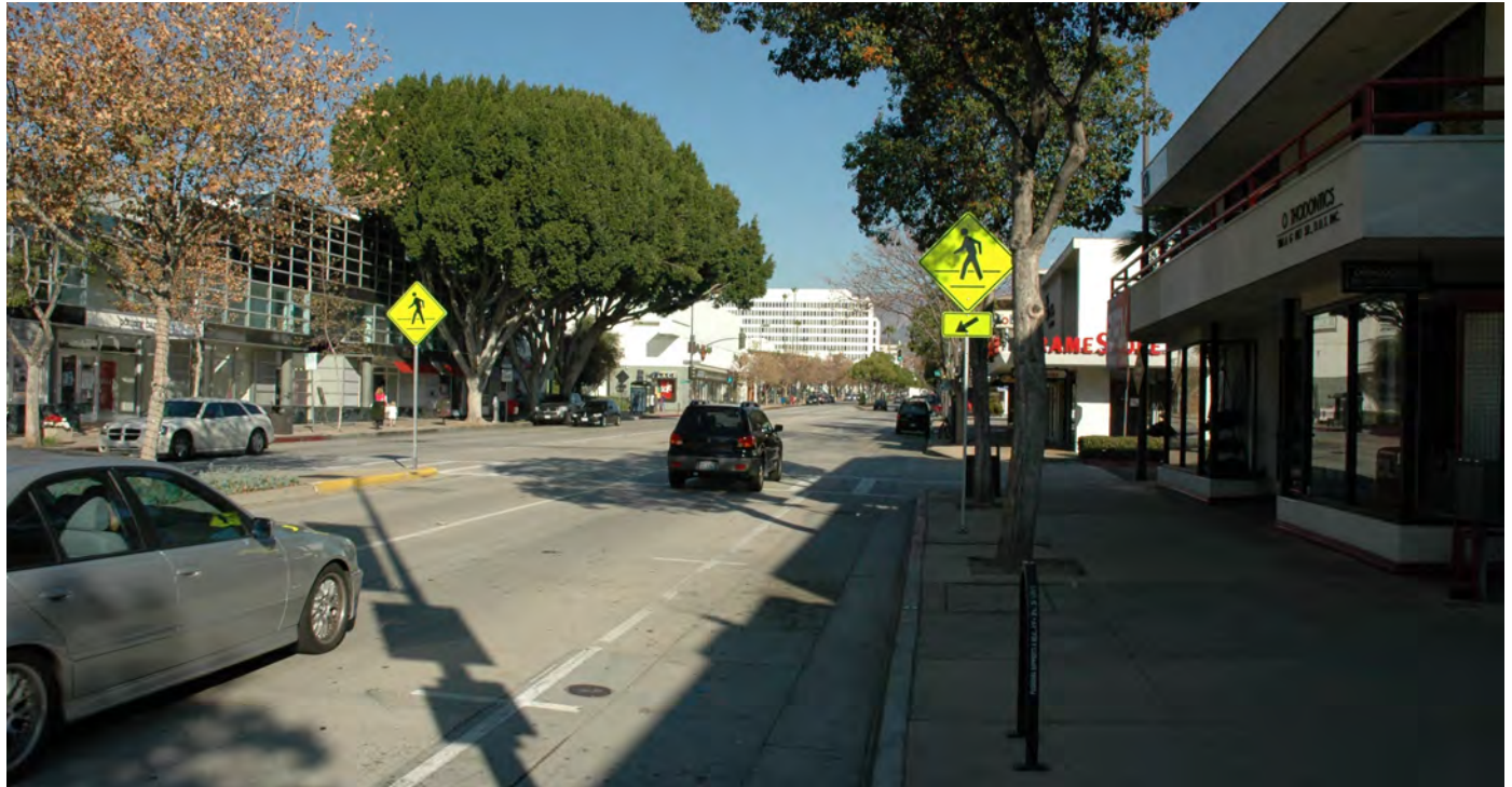
Lake Avenue in Pasadena, CA is a major north-south corridor which has two lanes of traffic in each direction, a planted median, on-street parallel parking, restaurants, retail and office with moderate to low density neighborhoods behind. This street is posted for 35 m.p.h. traffic.
