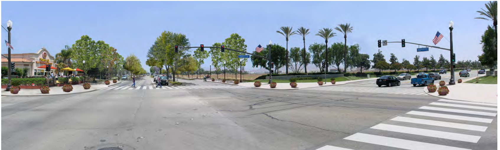
Above: Reconfiguration of Alessandro into two through lanes in each direction with frontage roads and curb extensions. The existing restaurant could extend its dining area on to a sidewalk patio.
