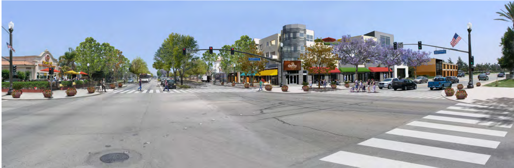
Alessandro Boulevard at Frederick Street showing varying degrees of change toward becoming the Civic Center Node
