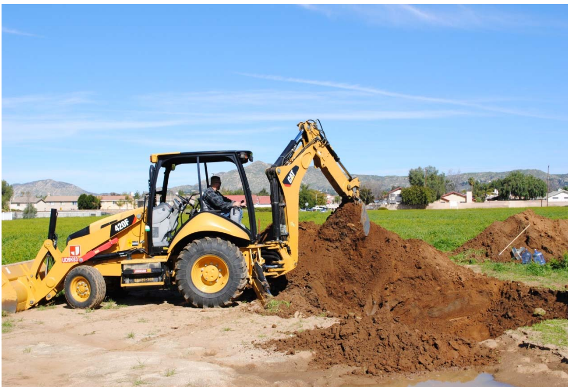
Photo 3 – Looking North at the Excavation for IT-8
