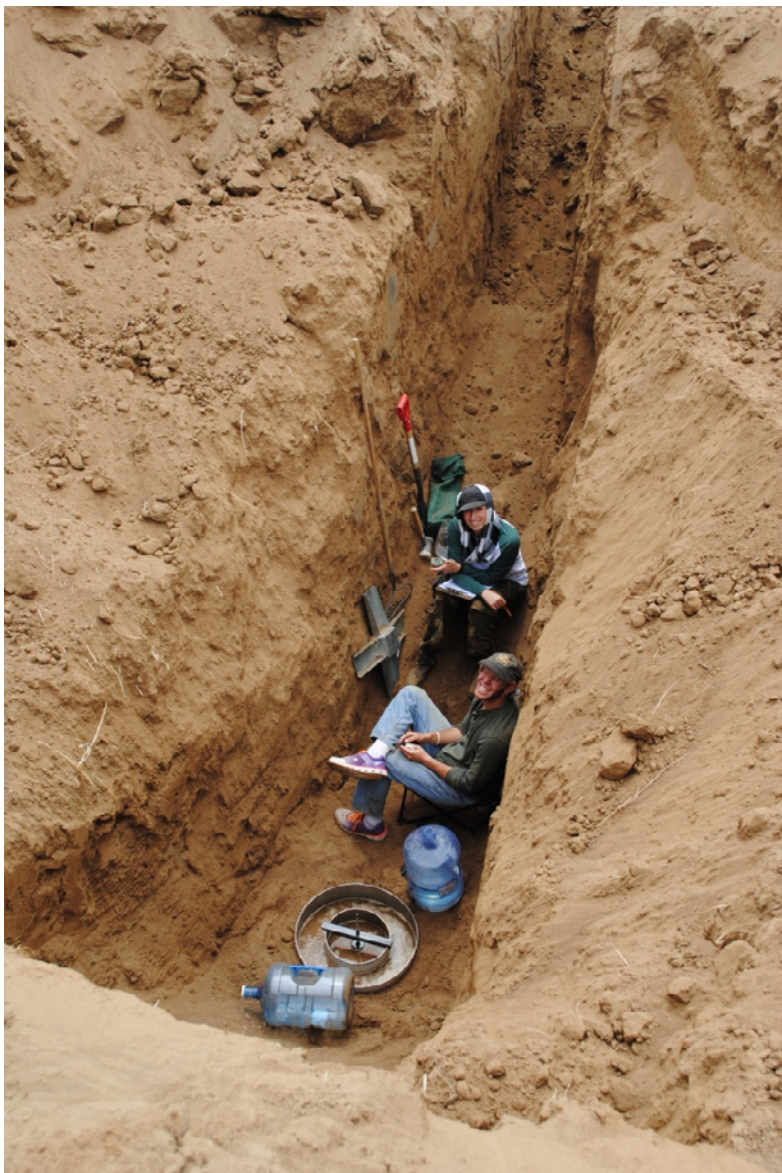
Photo 13 – Looking South at the Excavation and testing for IT-9
