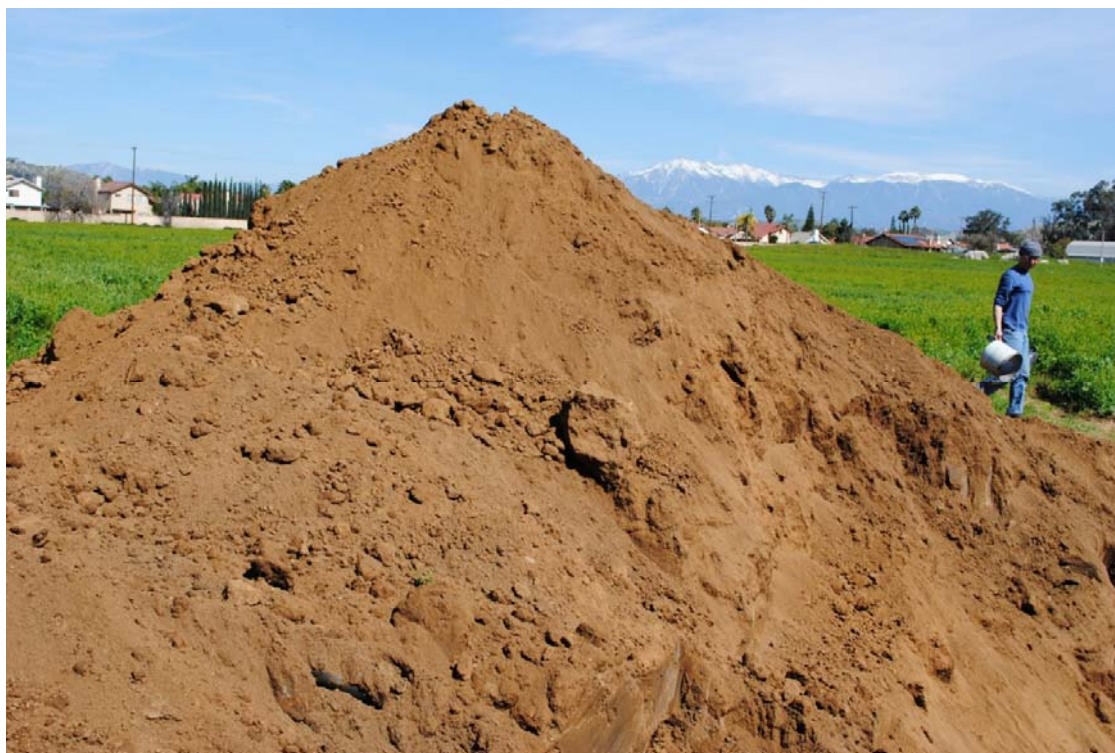
Photo 7 – Looking at the Excavated Soils from IT-8
