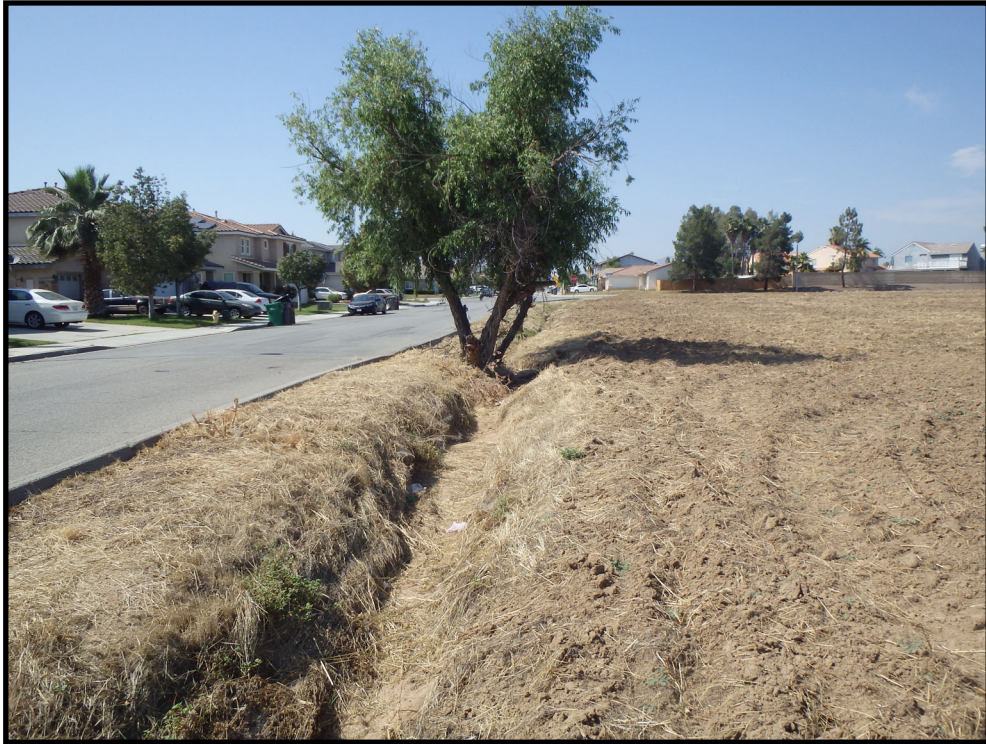
PHOTOGRAPH 1 - Looking upstream from downstream portion of AA1. Tarano Lane serves to confine flows along the western bank of the unnamed drainage.
