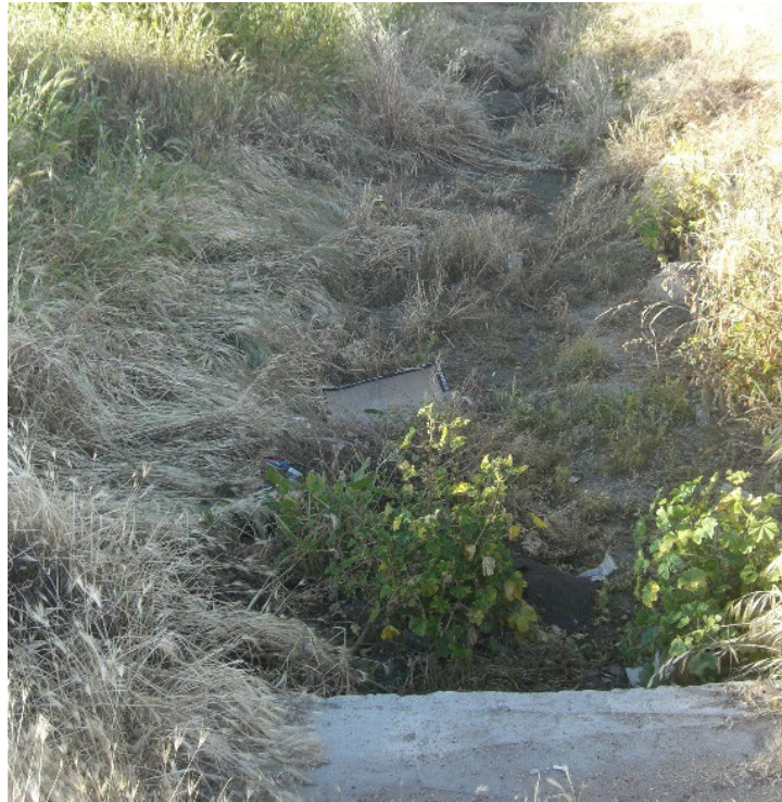
Photograph 6: Project Site's ephemeral drainage ditch, view towards the south
