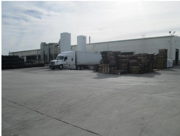
5. View of the Site from the southwest.
