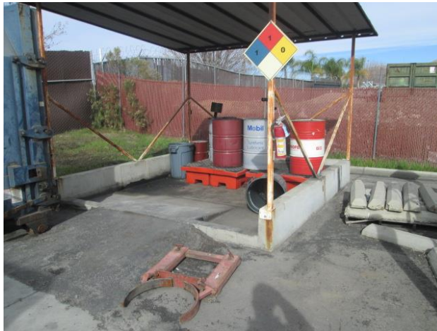
11. Used oil storage.
