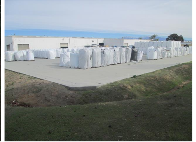
3. View of the Site from the southwest.
