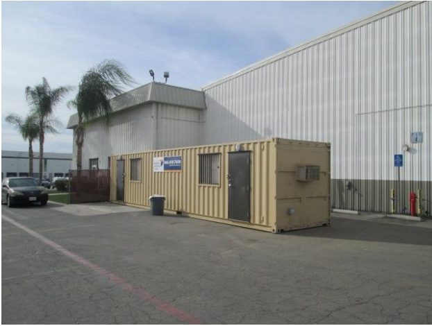
7. Eastern side of the Site building.
