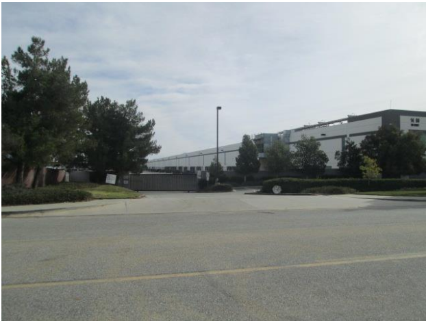
22. Southern adjacent property.
