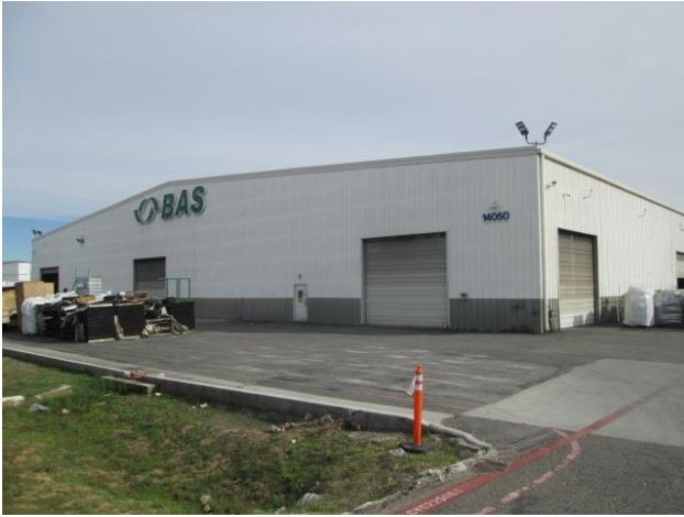
1. View of the Site building from the northeast.
